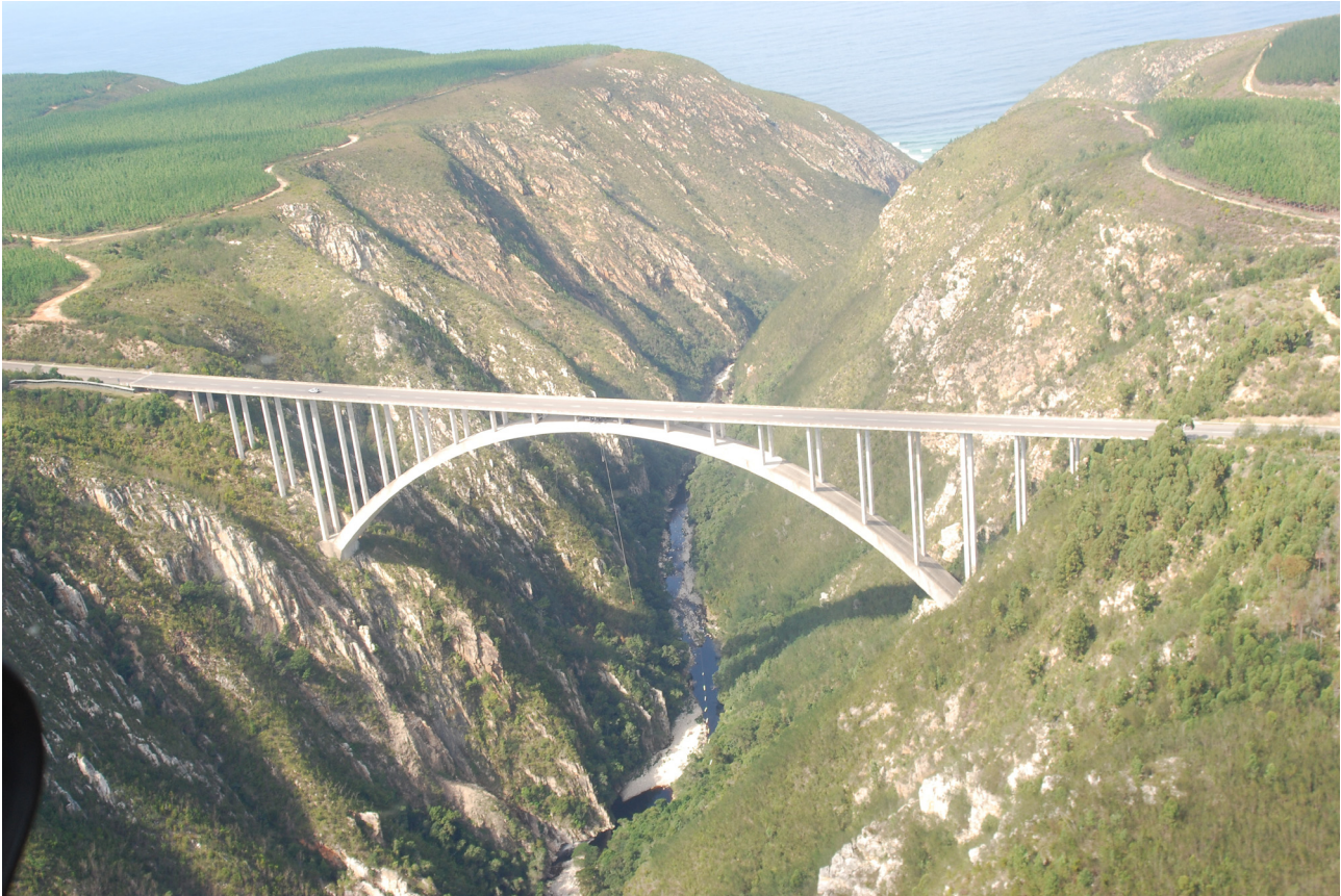
FIGURE 1. Deeply-incised gorge with bridge crossing the Bloukrans River, at the border of the Eastern Cape and Western Cape Provinces, South Africa. Photo F.C. de Moor.
