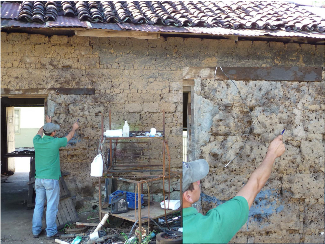
FIGURE 3. L. E. S. Martinez pointing at holes made by bees nesting in adobe wall in Bagaces.
